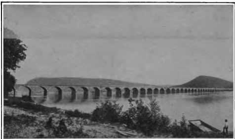
Rockville Bridge, Susquehanna River, west of Harrisburg.
