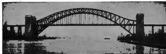
HELL GATE BRIDGE
