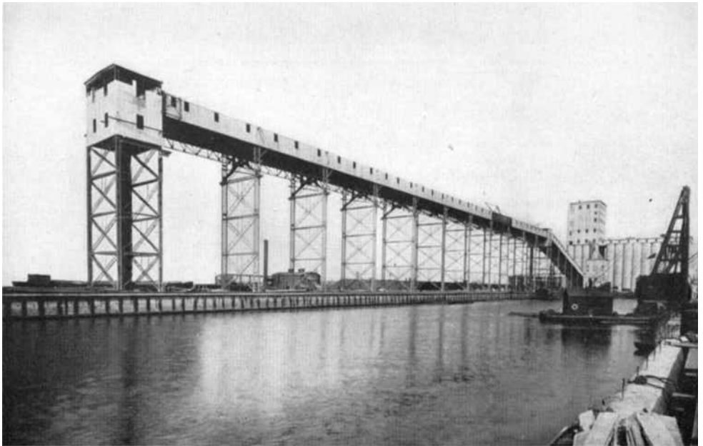
A MODERN FIREPROOF ELEVATOR FOR HANDLING EXPORT GRAIN AT PHILADELPHIA Grain from the Great Lakes, which comes to Philadelphia from Buffalo and Erie, is handled here.
