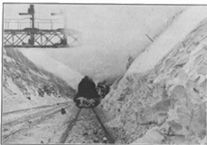
Cut Approaching the Westbound Tunnel near Gallitzin—Drifts 15 ft. Deep
