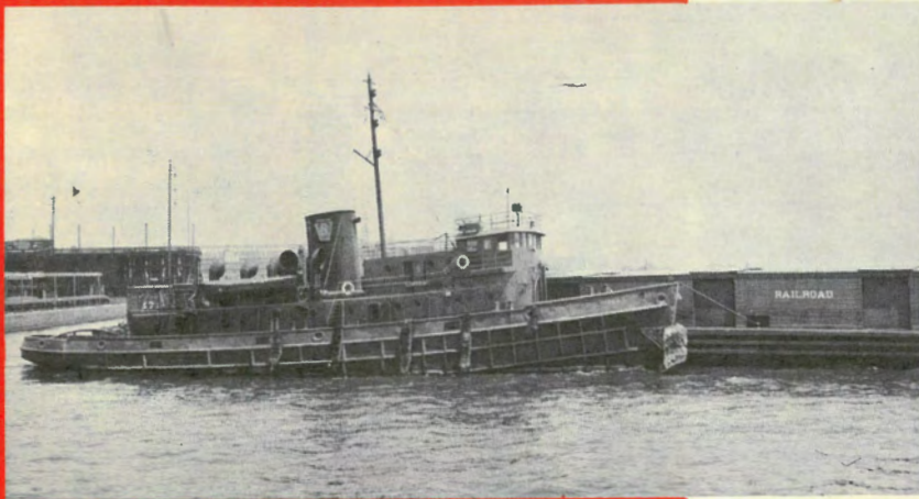
A LEADER of Pennsylvania's fleet of 30 tugs in New York Harbor, the 140-foot LINDEN, with radio-telephone and fire-fighting equipment, has an oil fired engine developing 1,200 horsepower. Built in 1944 for the U. S. Army, it was used in World War II in European waters, having crossed the Atlantic Ocean under its own power.
