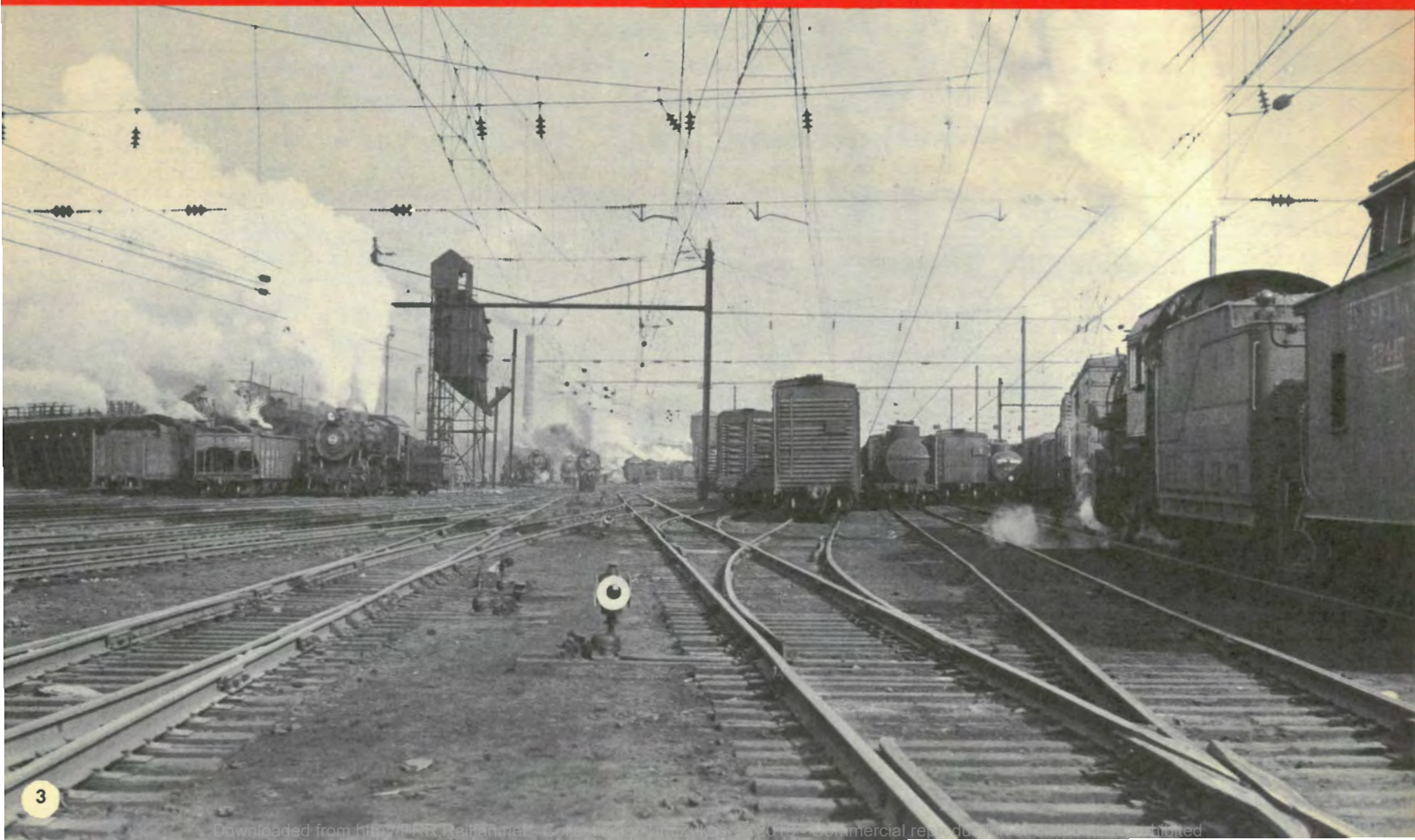
▼ MEADOWS YARD , capacity 5,484 cars, serves as a supporting yard to Harsimus Cove where export cars are classified for movement to shipside by carfloat or lighter and where import cars are classified for interior destinations.
