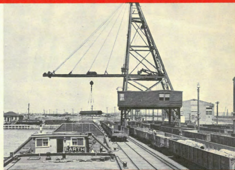
ONE OF FOUR traveling gantry cranes on Pier B, Greenville, transferring export freight from cars to lighters.
