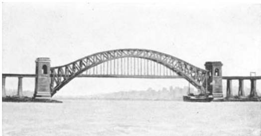
Hell Gate Bridge
