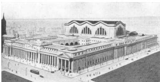
Pennsylvania Station, New York City
