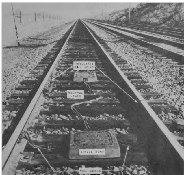
Figure 2 Impedance Bonds
