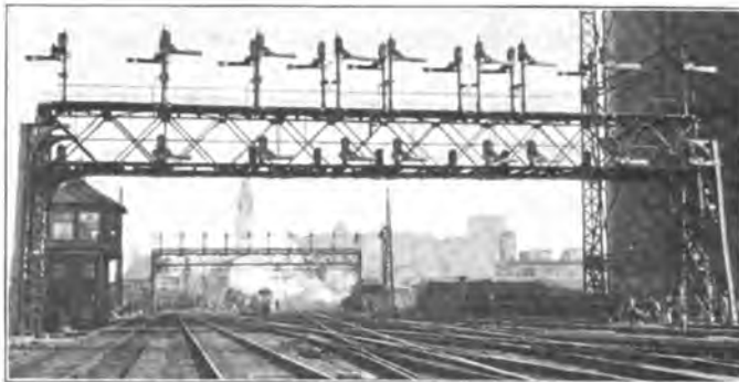
Erecting New Signal Bridge Around the Old One in Busy Terminal.
