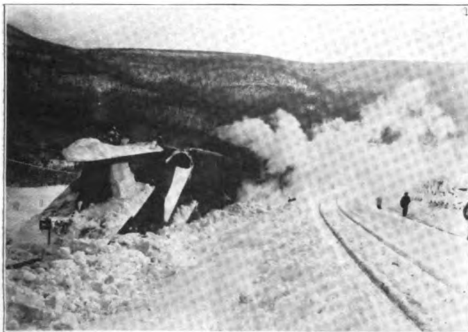
Fig. 1. Snow Plow and Three Pusher Locomotives Starting Out to Open Up the Line.
