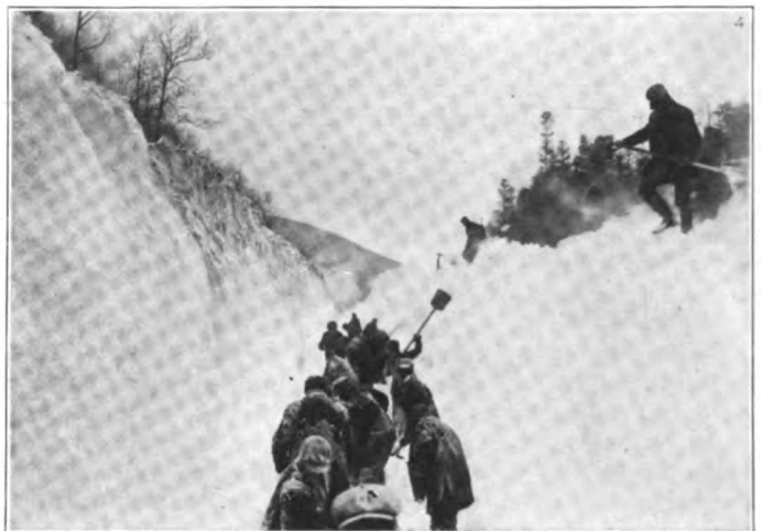
Fig. 4. Cut Made Through Deep Snow After Plow Had Passed Through. Men at Work Shoveling Out a Flangeway.
