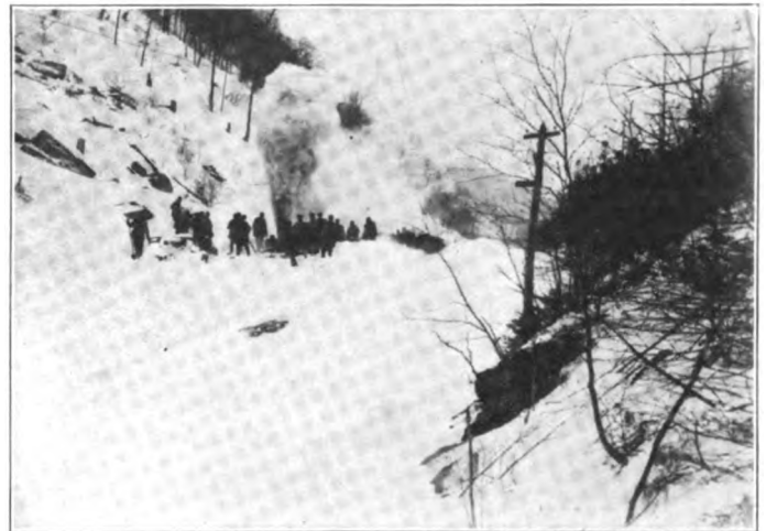
Fig. 3. Three Engines Pulling in a Train, and Unsuccessful Attempt to Extricate Plow. Cupola of Plow Only to Be Seen in the Picture.
