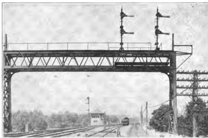
One of the Signal Bridges at the East End of the Plant.
