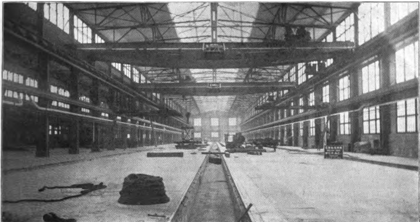
Erecting Shop, Showing Two 75-Ton Girder Cranes and Three Traveling Wall Cranes, Havelock Shops.
