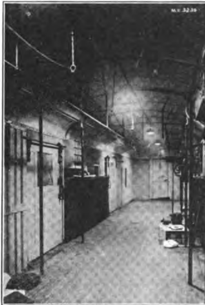
Fig. 1. Present Spacing Using BAD-60 Holophane Reflectors. Note the Heavy Shadow Lines Between the Units on the Upper Walls.
