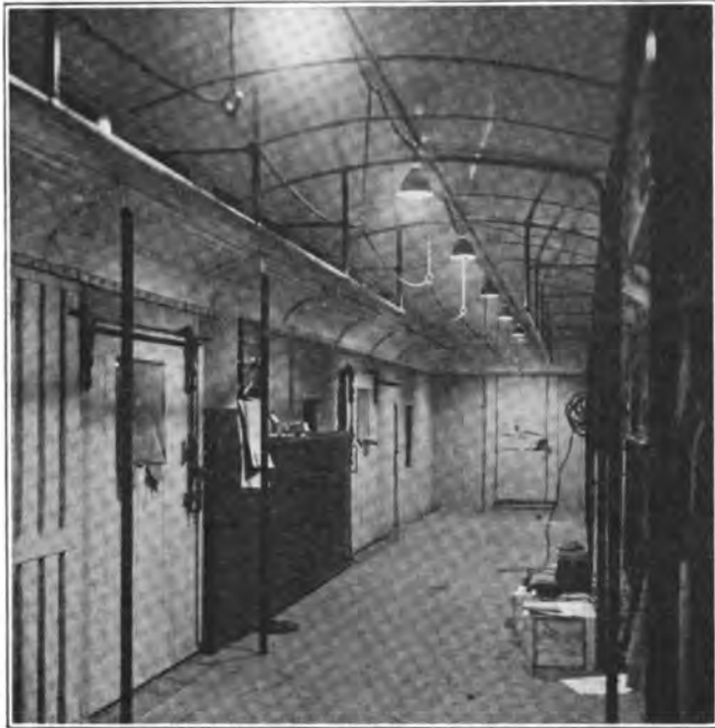
Fig. 4. Showing the Illumination with Deep Bowl Reflectors. Holophane No. 18460. Notice that Rather Heavy Shadows Are Cast on the Side Walls and Upper Ceiling Due to the Screening Angle of the Reflector.
