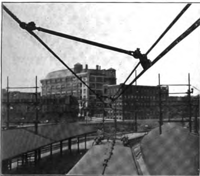
Fig. 10. Non-Corrodible Tube Trolley Hanger.
