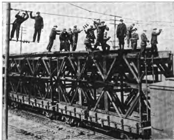
Fig. 11. Special Car for Erecting Catenary Work; Removable Outriggers Make It Possible to Work Over Adjacent Track Without Interruption to Traffic.
