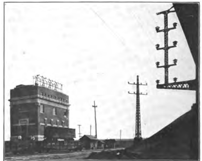
Fig. 4. View of the West Philadelphia Substation Showing Entrance of the Four Single-Phase 44,000-Volt Lines from the Arsenal Bridge Substation. The Method of Carrying These Lines on the Elevated Structure is Clearly Shown at the Extreme Right.
