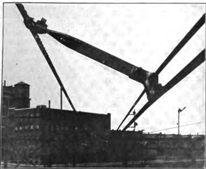
Fig. 9. Wrought Iron Trolley Hanger and Method of Its Attachment to the Wires in Curved Track Construction.
