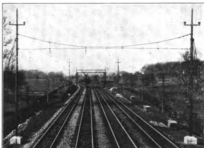
Fig. 6. Tubular Cross-Catenary Bridge Before Longitudinal Wires Were Erected.
