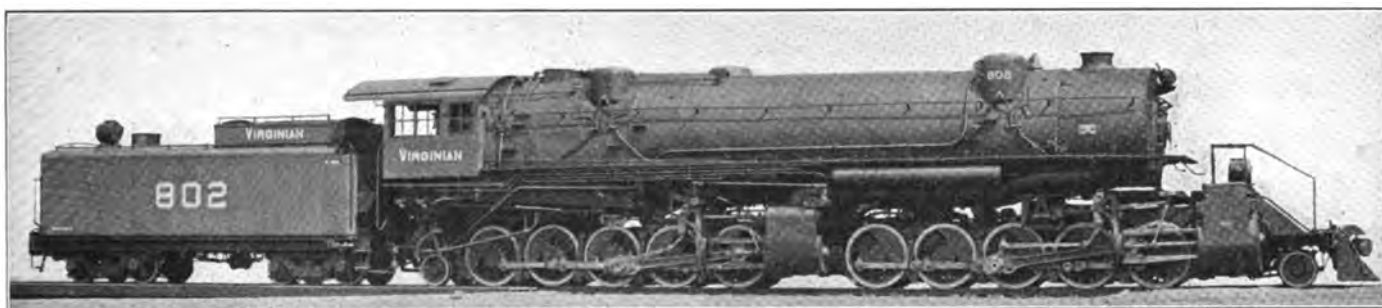
Virginian 2-10-10-2 Type, the Most Powerful Locomotive in the World
