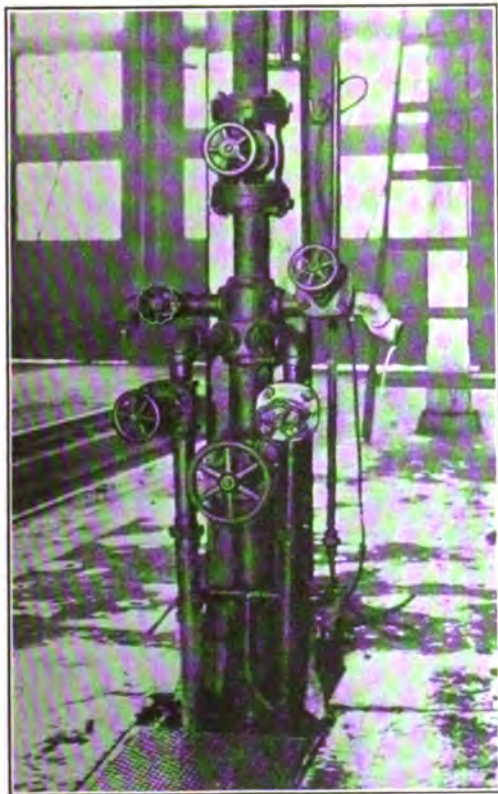
HOT WATER WASHOUT SYSTEM, MANIFOLD PIPE LINES IN CONDUIT.
