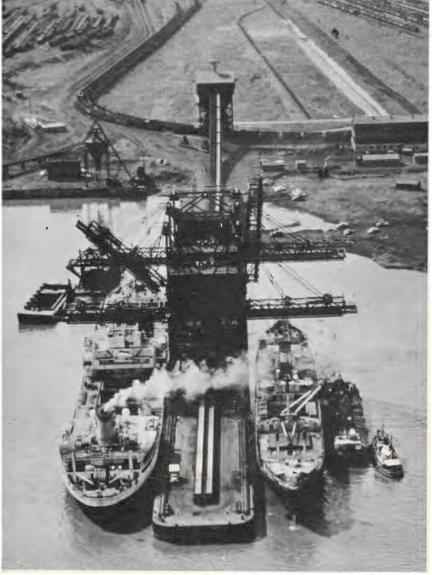
Two cargoes of import ore being unloaded simultaneously at the new Greenwich Point Ore Pier, in Philadelphia.
