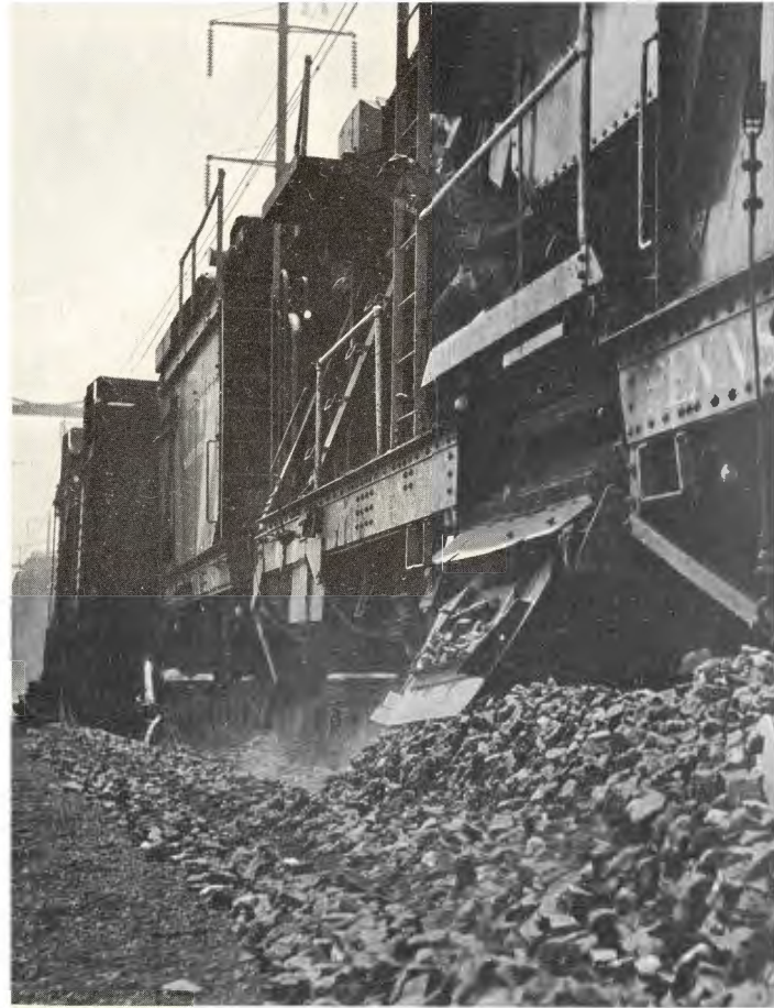
More than half of all work on track maintenance is now done mechanically, with substantial economies. This Brownhoist ballast cleaner is operated by only eight men.
